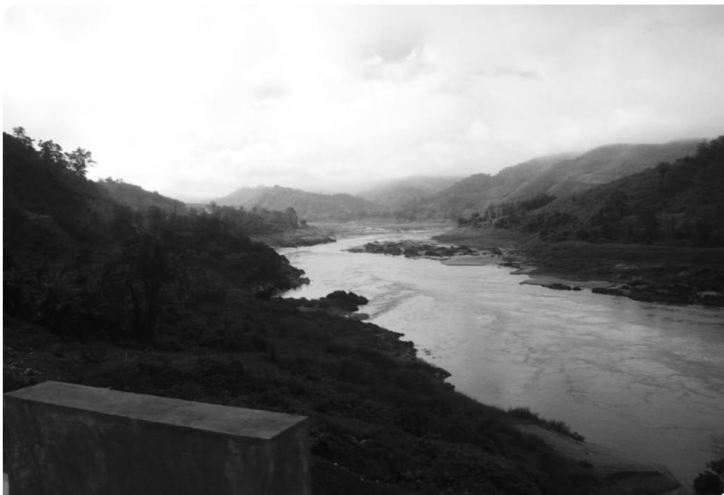
ABOVE: Site of the future Pak Beng Dam.
